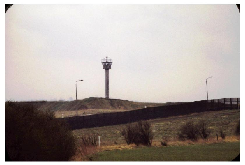
The new tower was a pre-fabricated structure that took three days to build once the foundation was set. In all towers, as in all patrols and movements, were two men (usually one married and one single) to watch each other.
